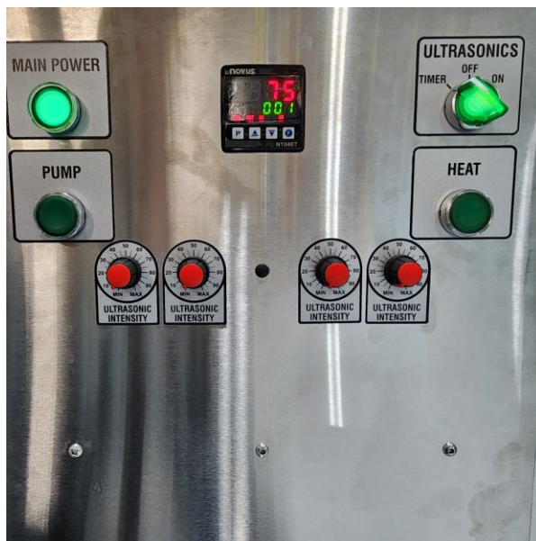
Figure 15: Generator Timer Running
