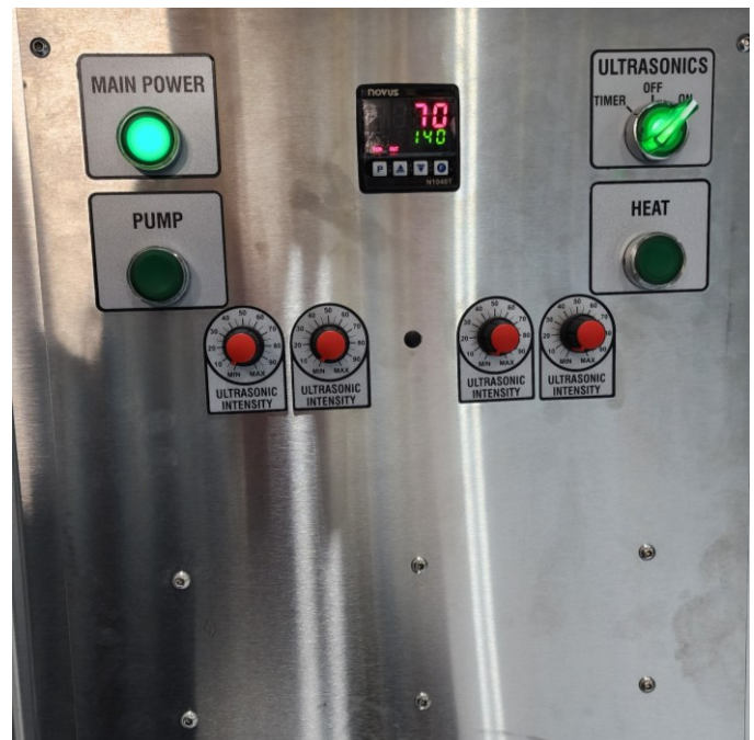
Figure 11: Generator Manual Control On
