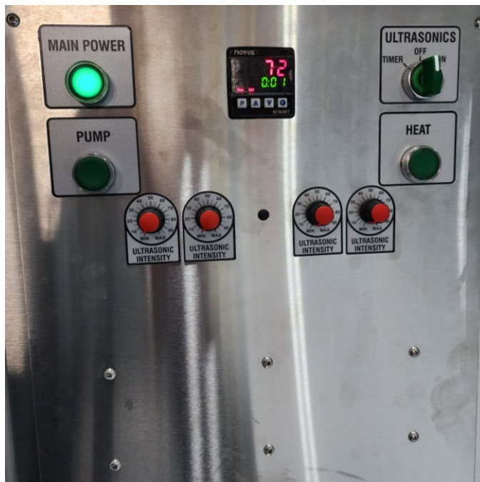
Figure 10: Generators Manual Control Off
